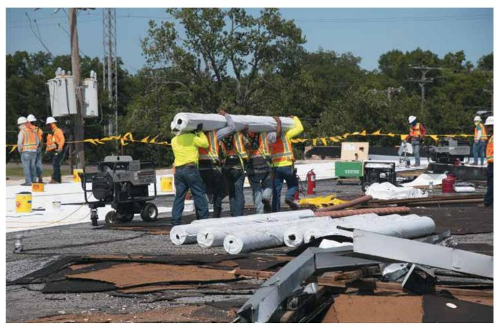
Figure 7. Five workers lifting and transporting a roll weighing over 400 lb (180 kg).
