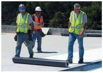
Figure 4. Worker laying out roof roll.
